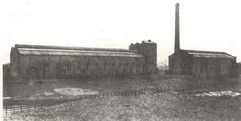
VIEW OF HOLLINWOOD WORKS IN 1896
