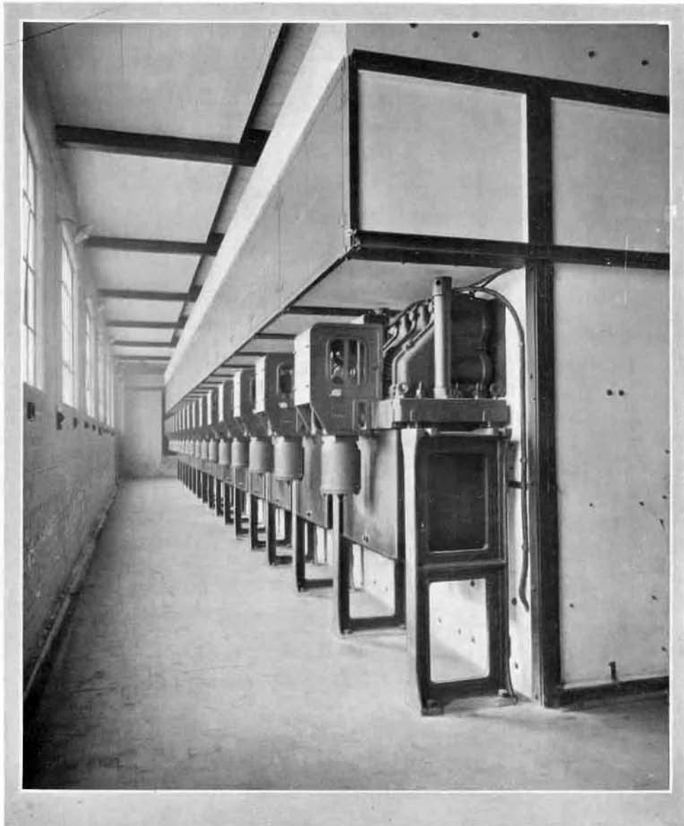
INTERIOR OF SWITCH HOUSE, WITH REMOTE CONTROL SWITCHGEAR
