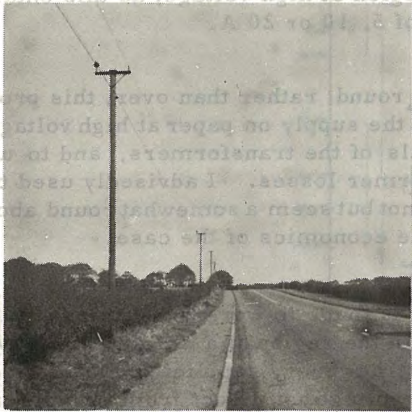
SINGLE PHASE 6.6kv LINE NEAR NORTHWICH
