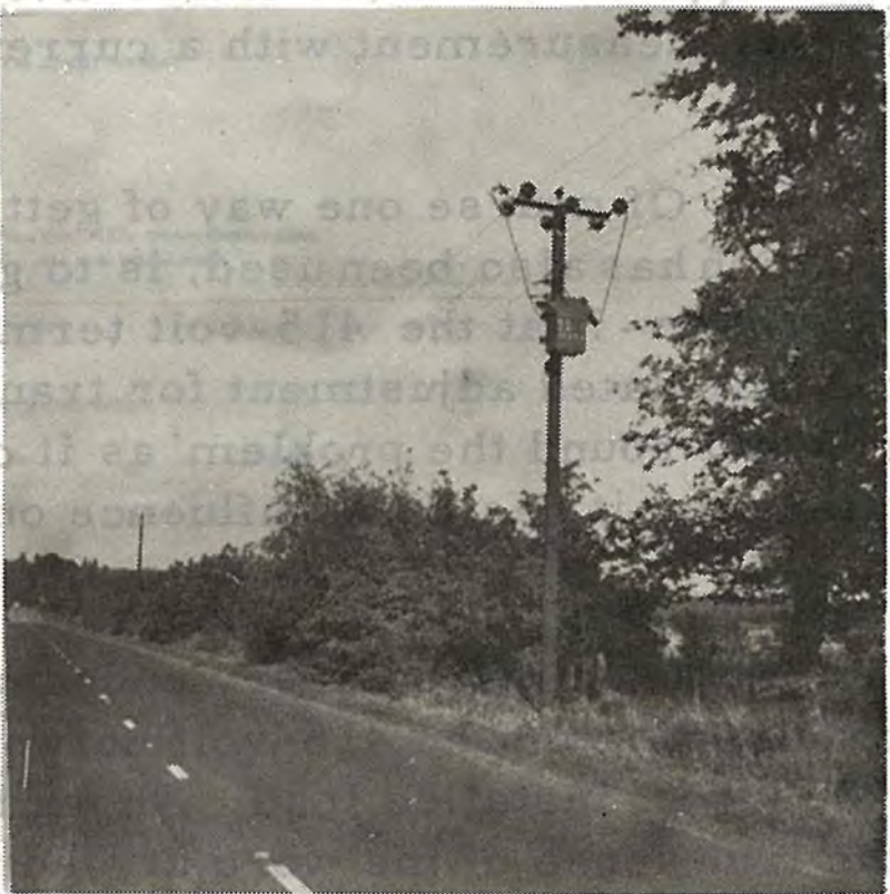
10 kVA TRANSFORMER - NEAR NORTHWICH
