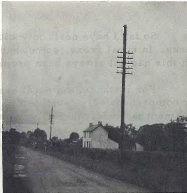
COMBINED 415 VOLT AND TELEPHONE LINE
