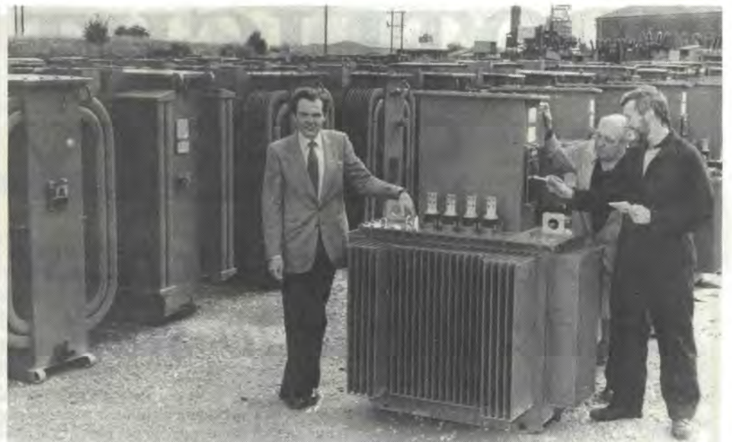
Chargehand Ken Palframan checks in the new corrugated transformer with colleague Bob Wynn, right, watched by the author, Geoff Wood. The transformers to the left are the same capacity as the small corrugated one in the foreground, but are physically much larger.
