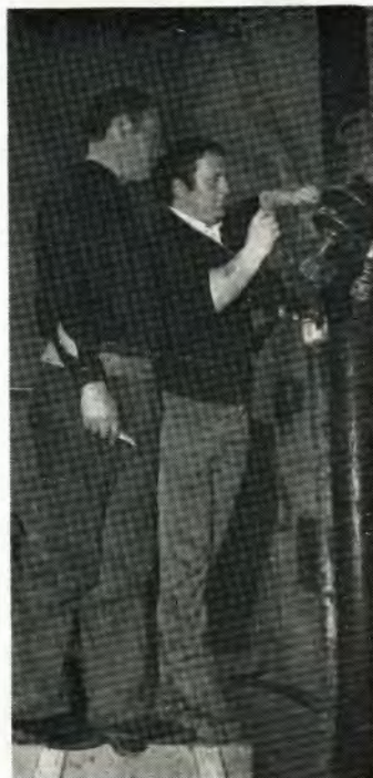
Mr. M. Lavelle (North Wirral) with his mate, Mr. T. Male making off an 11,000 volt pole box.
