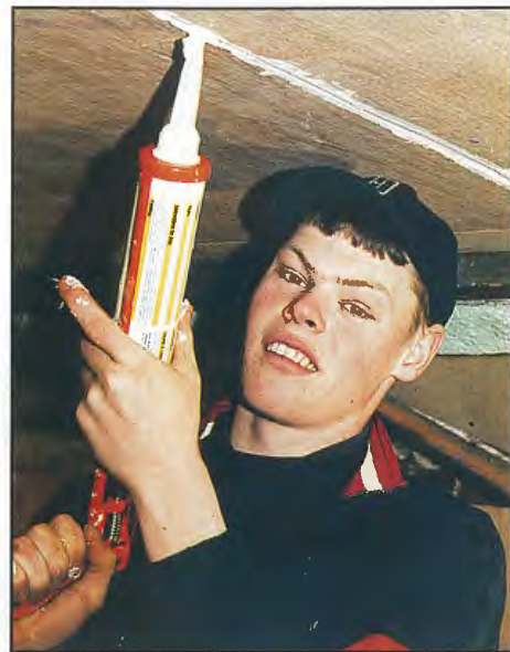
Trust Volunteer Nathan Thomas, aged 17, filling gaps in the toy room ceiling.
