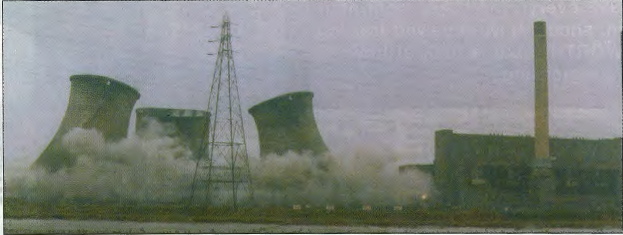
Sheer dynamite! The towers are reduced to rubble in a matter of seconds.
