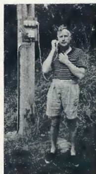
While on holiday last summer on a camp site in Southern Brittany, Mr. Speaight takes time out for a shave by plugging in his electric razor to a socket outlet mounted on a lighting pole.
