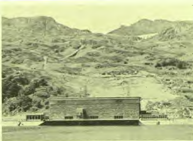
Fig. 15. Ffestiniog Power Station—pumped storage scheme—with Stwlan dam 1000 feet above.
