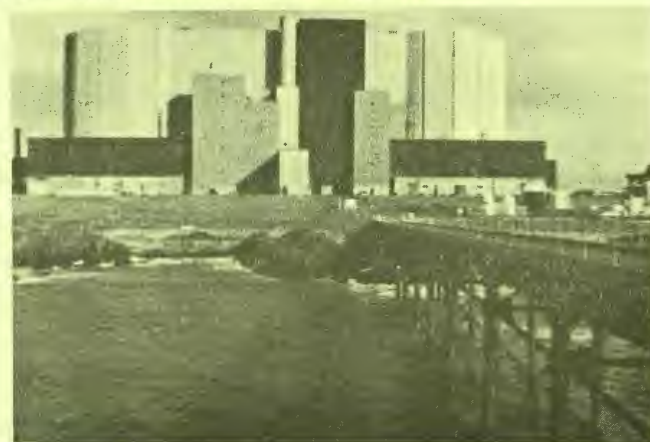
Fig. 17. Reactor building at the Wylfa nuclear power station.
