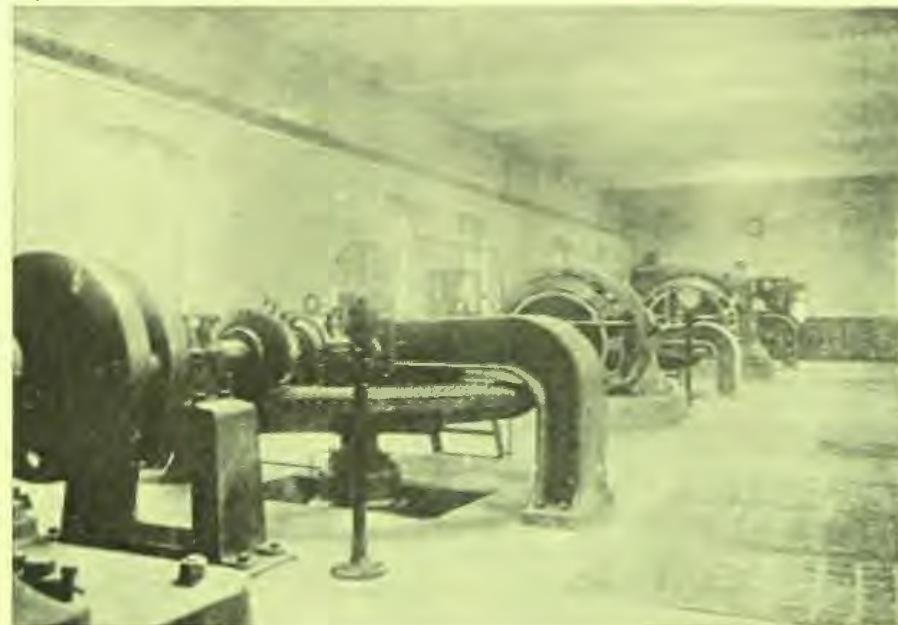
Fig. 13. Hydro Works, Chester, 1913.
