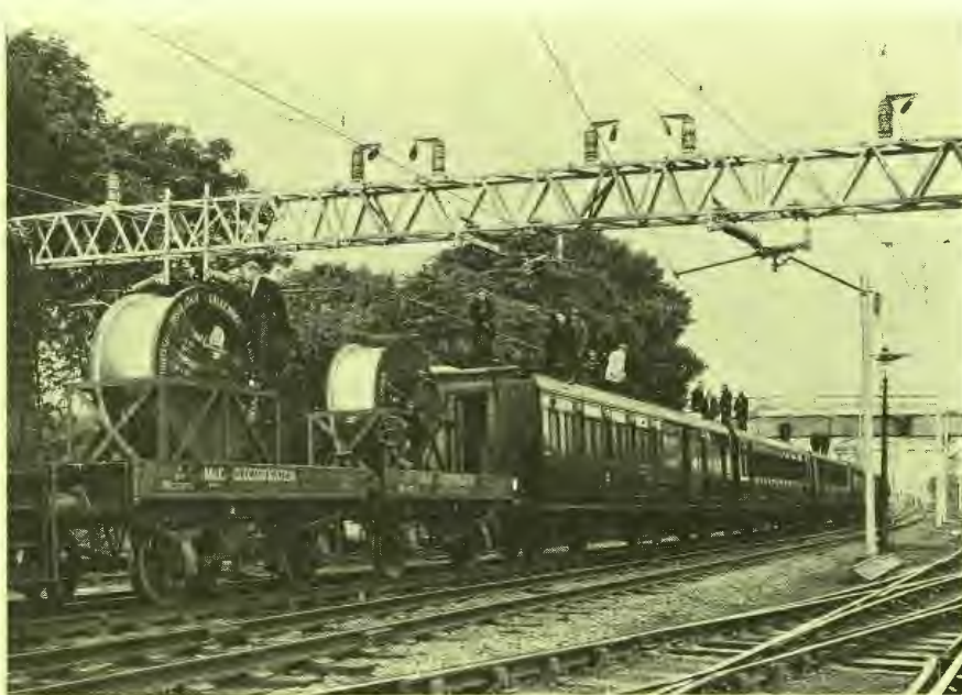
Fig. 7. London Midland rail electrification—running contact wire at Wilmslow.
