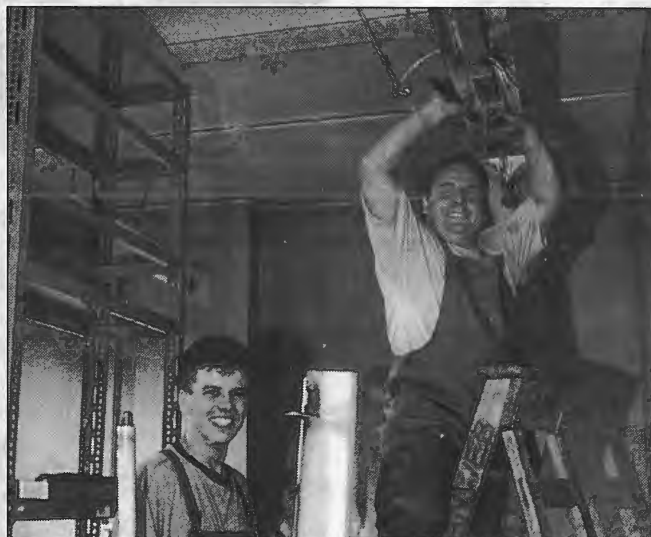
Electricians Paul Owens and Dave Loyley at work on the Vulcan Street site.
