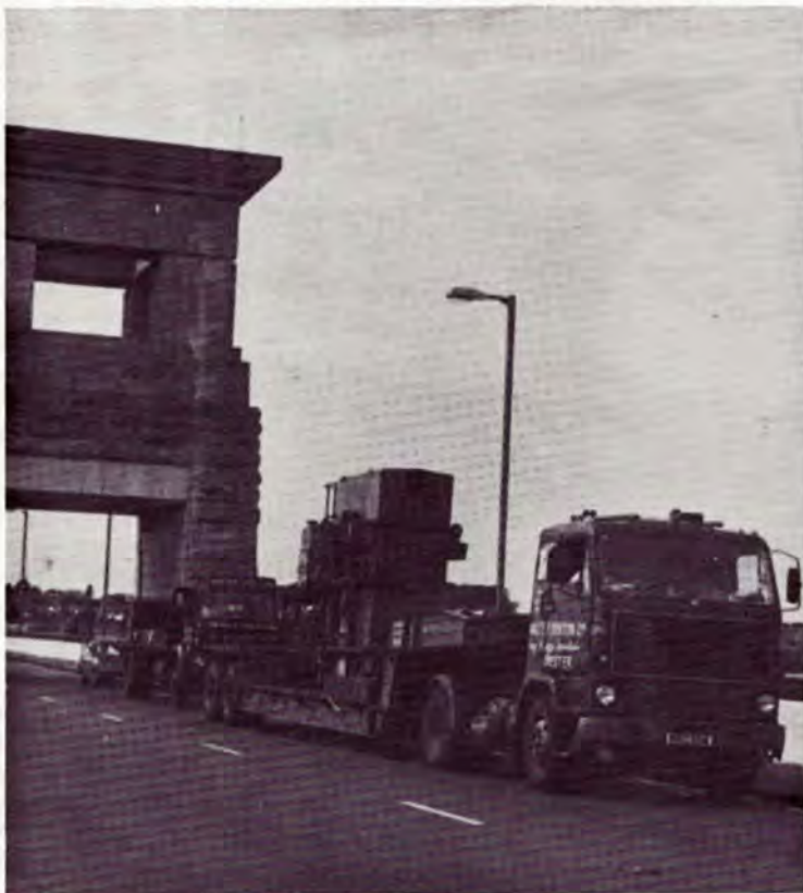
The 27-ton transformer being transported across the new road deck.
