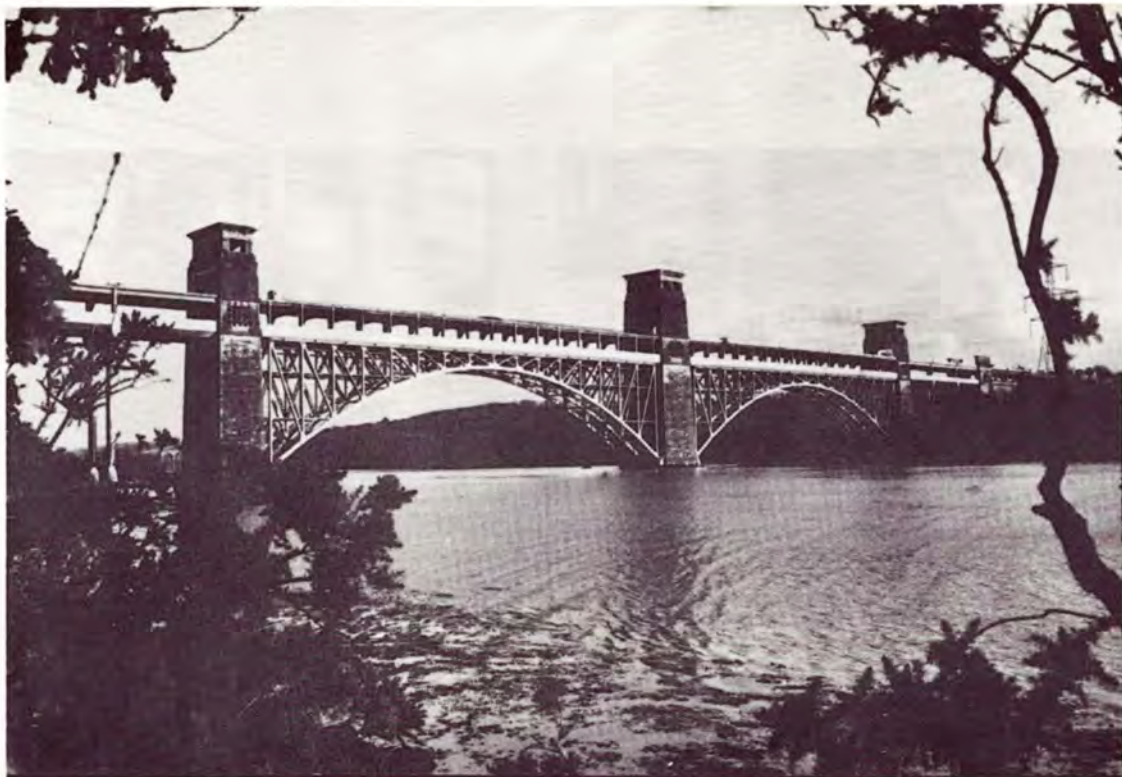
The impressive Britannia Bridge with the new road deck built above the railway track.
