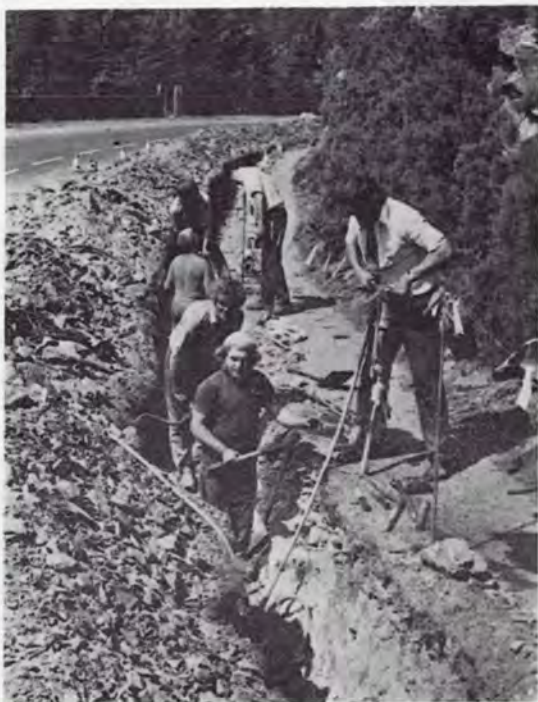
These pictures explain, better than any words, why it would not be practical to underground all electricity supplies! This trench, along the main road near Llanberis, will carry a 33kV cable replacing overhead supplies which are being diverted to allow work to go forward.
