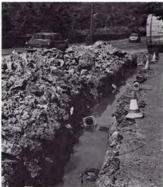
These pictures explain, better than any words, why it would not be practical to underground all electricity supplies! This trench, along the main road near Llanberis, will carry a 33kV cable replacing overhead supplies which are being diverted to allow work to go forward.
