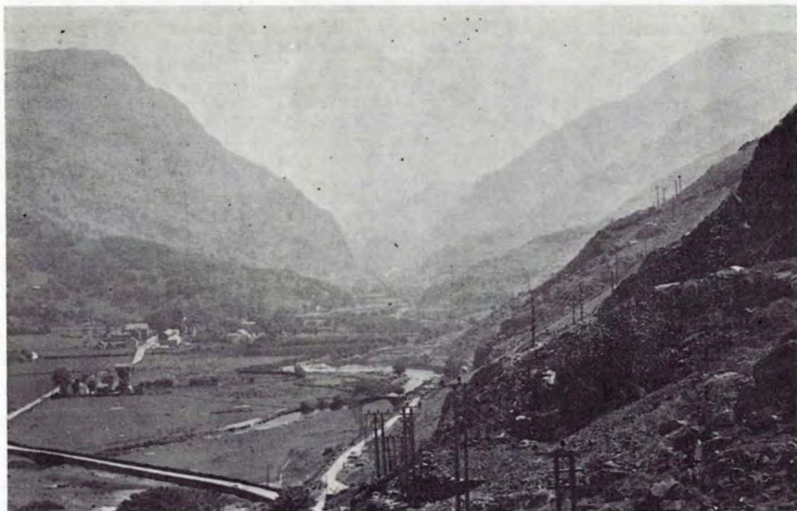
The line being dismantled can be seen descending into the valley, while the new lines replacing it march over the hillside on the right.
