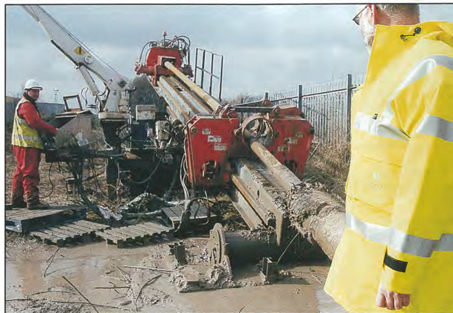
The Trenchless Technology "mole" is fired up and ready to go.
