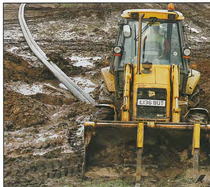
The experts prepare to insert the cable into the pipe
