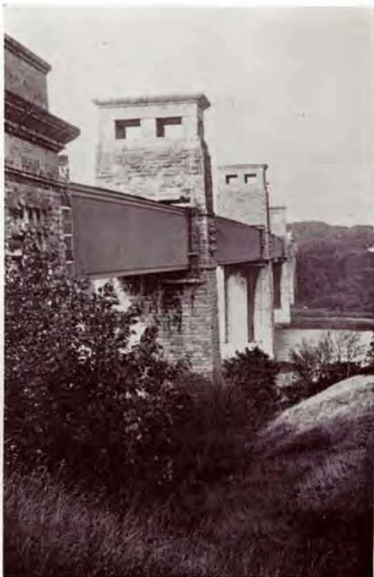
Britannia Bridge, linking Caernarvon with Anglesey, where MANWEB engineers recently carried out 'cable lifting' operations.
